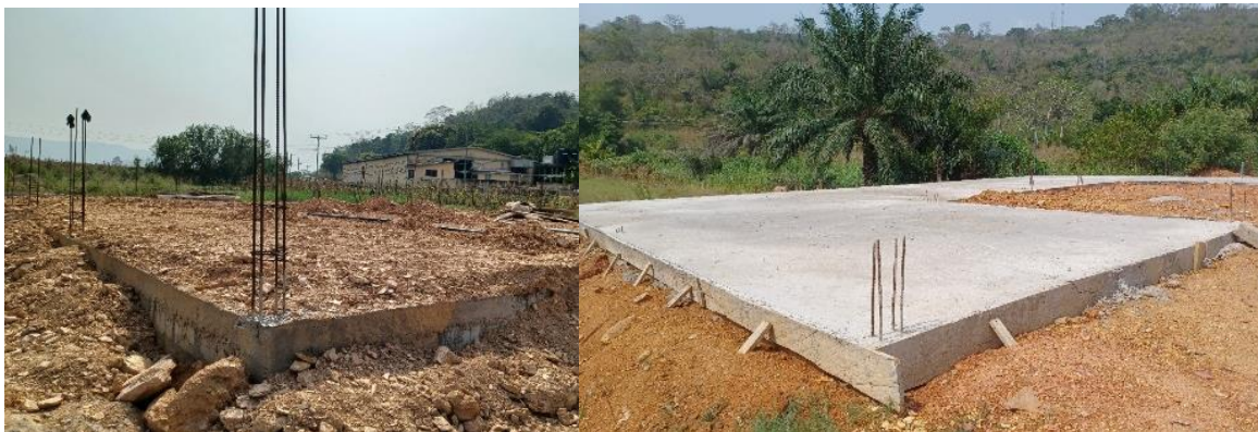
Figure 3.1.1: Ecohub structure at various stages of construction for Pre-fab installations.
