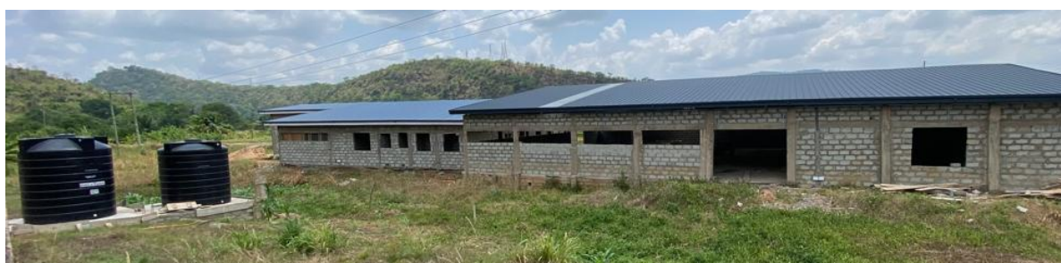
Figure 3.1.6: Innoecofood project Ecohub indicating the fish hatchery, fish processing structure, and mechanised borehole water systems under construction at CSIR-WRI, ARDEC, Ghana.
