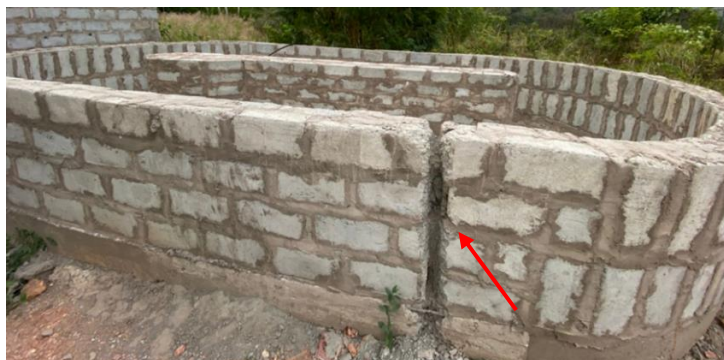
Figure 3.1.7: Inlet and outlet pipe installation works for Spirulina pond.
